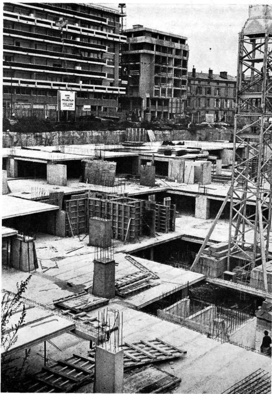
Construction du parking Saint-Georges.
